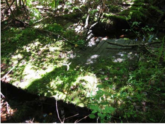
Footbridge over stream
