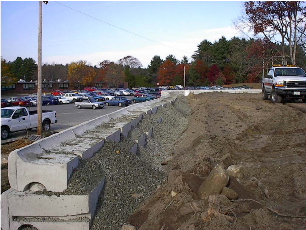
Athletic Field Retaining Wall Construction
