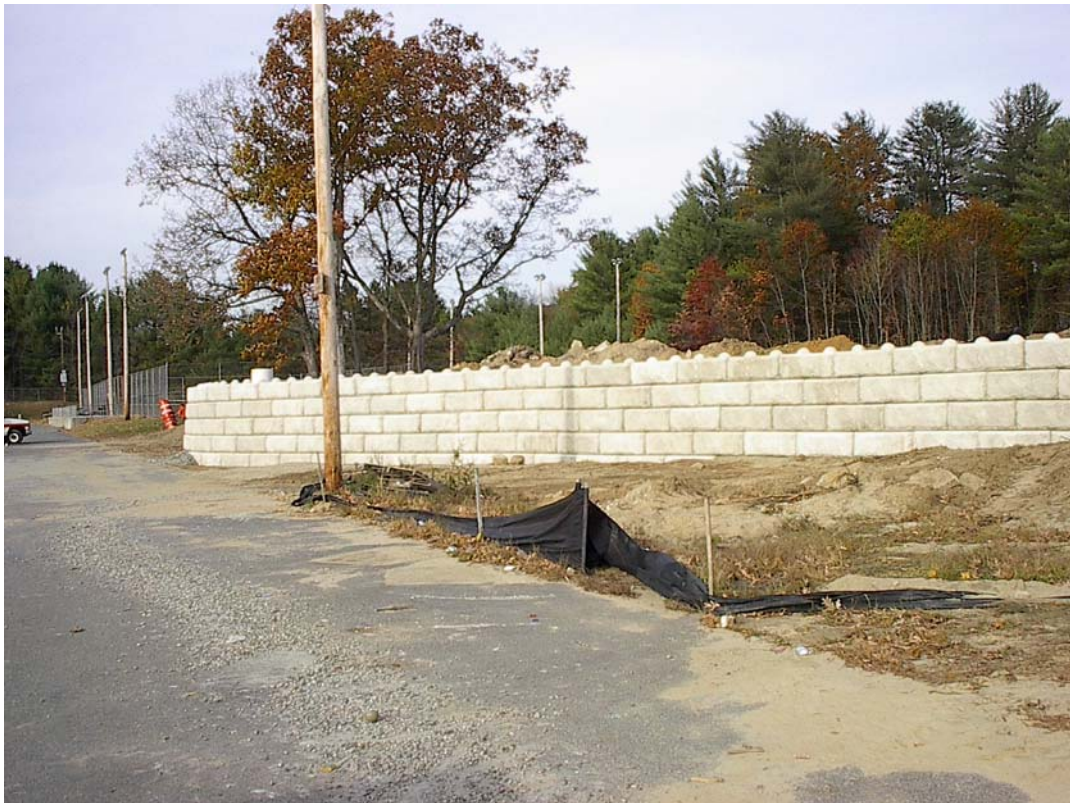
Athletic Field Retaining Wall Construction
