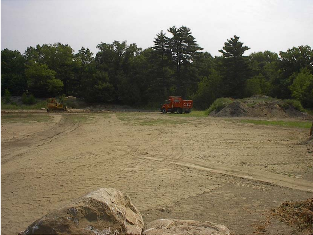
High School Athletic Field-Land Clearing Stage
