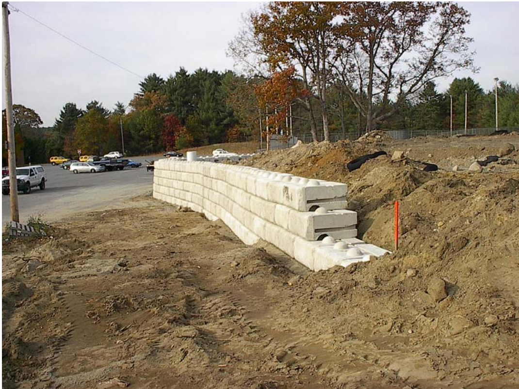
Athletic Field Retaining Wall Construction
