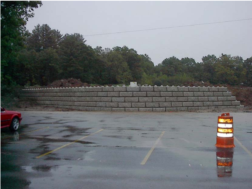
Athletic Field Retaining Wall Construction
