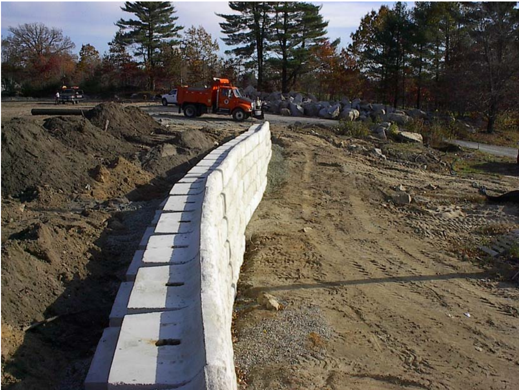
Athletic Field Retaining Wall Construction
