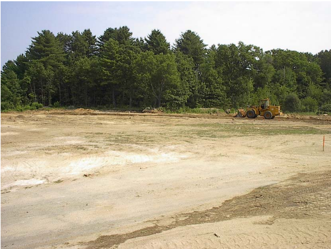
High School Athletic Field-Site Preparation Stage
