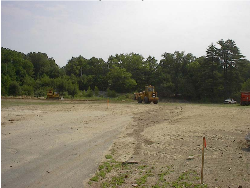
High School Athletic Field-Land Clearing Stage
