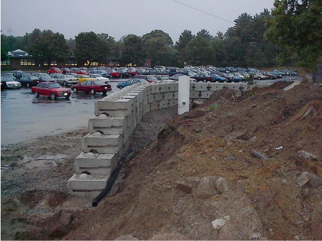
Athletic Field Retaining Wall Construction
