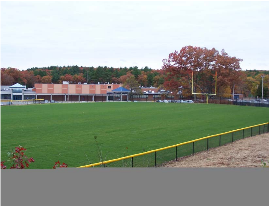
Athletic Field at 80% Completion
