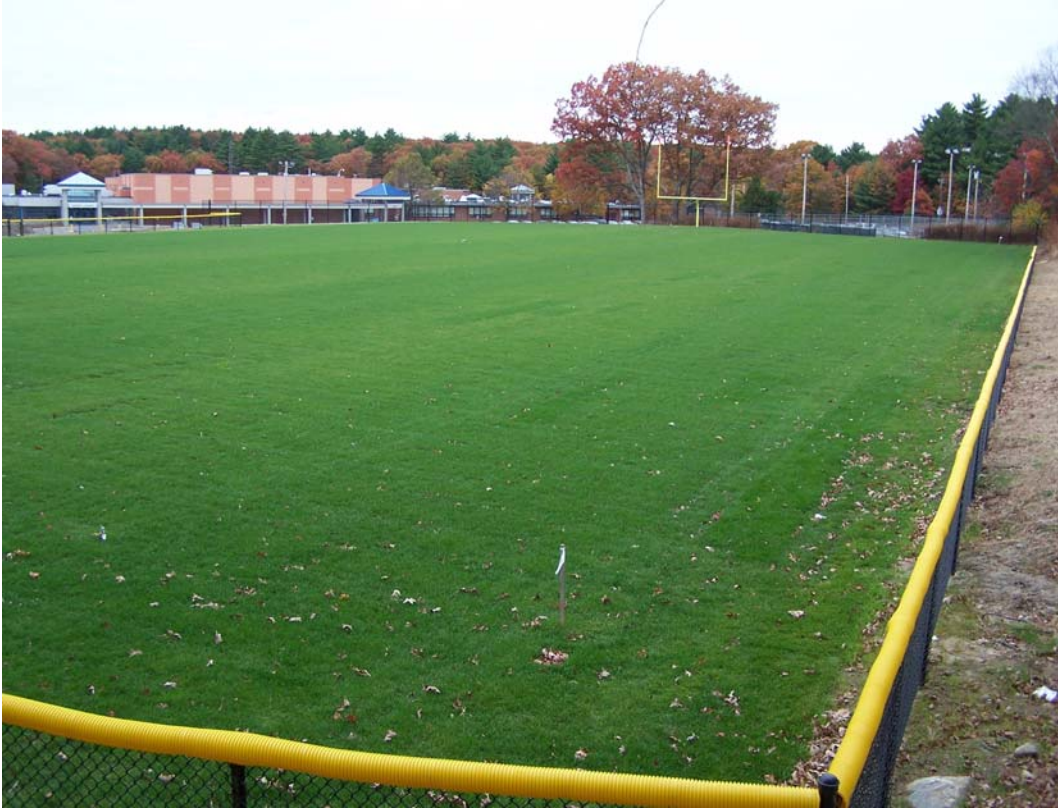
Athletic Field at 80% Completion
