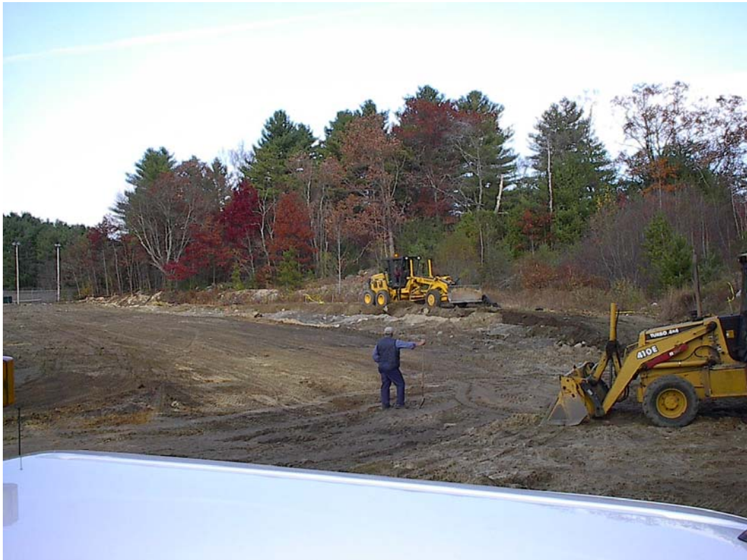
Athletic Field Site Excavations
