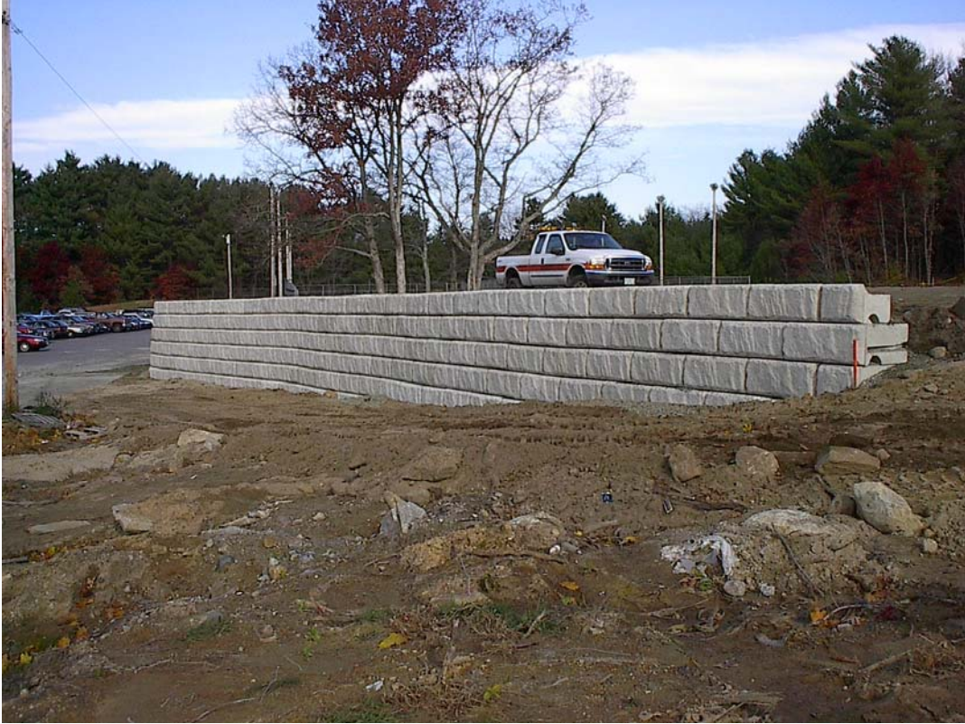
Athletic Field Retaining Wall Construction
