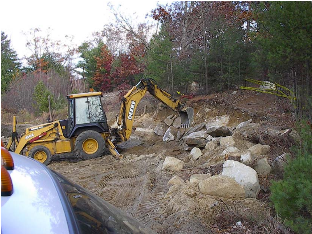
Athletic Field Boulder Retaining Wall Construction
