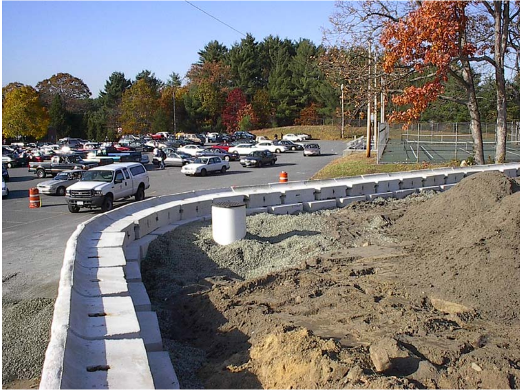
Athletic Field Retaining Wall Construction
