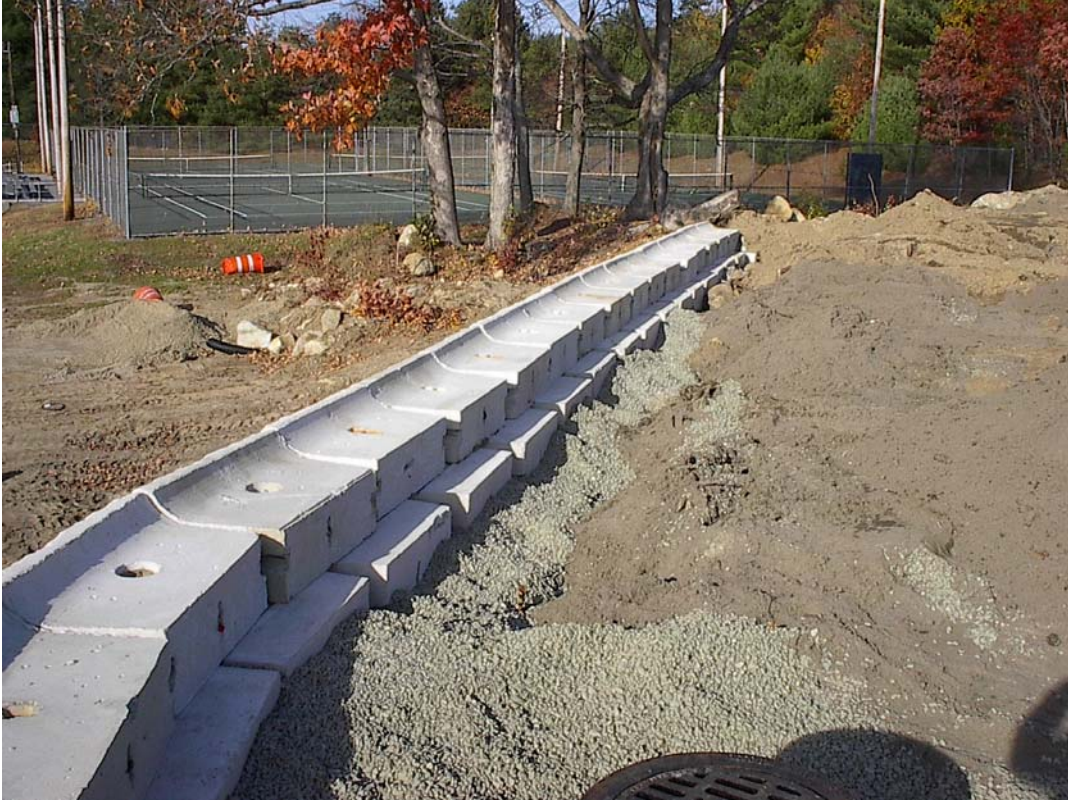
Athletic Field Retaining Wall Construction
