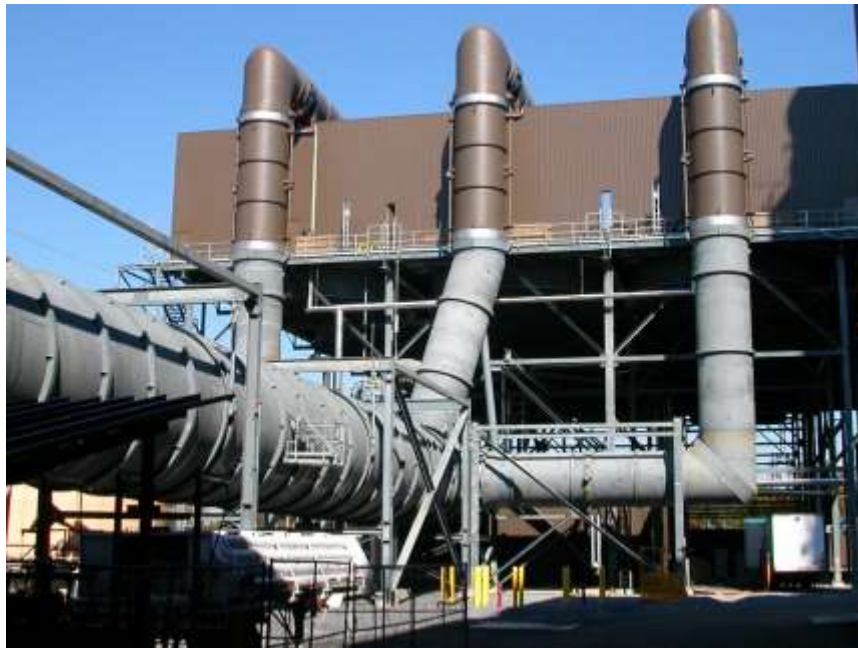
Figure 2 Typical ACC Steam Duct
