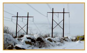
The proposed new transmission line will consist of approximately 57 new steel structures in the right-of-way. The structures on the south side would be "H" frame structures, approximately 85 feet tall, similar to existing structures along the right-of-way, and the structures west of the Clear River would be monopoles, approximately 110 feet tall.
